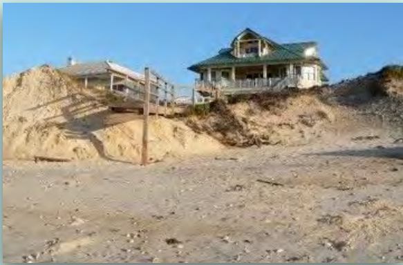
Erosion caused by Hurricane Dennis in 2005
