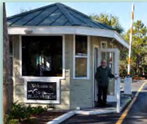
New guardhouse and entry gate
